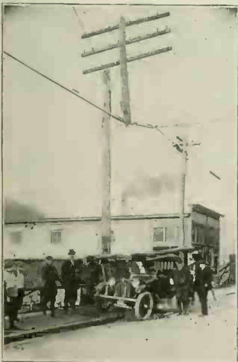
A Peculiar Accident In Which a Telephone Pole Was Severed By An Auto Crashing Into It. The Pole Remained Suspended By Its Own Wires.
