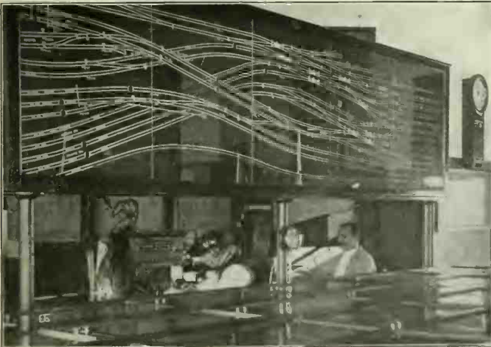
The Twentieth Century Railroad Tower Director Is a Very Important Personage Indeed. To Facilitate the Accurate Handling of Trains in Complicated Terminal Yards, Electrical Tally-boards Are Provided Which Show the Exact Position of Every Train by Means of Lamps.
